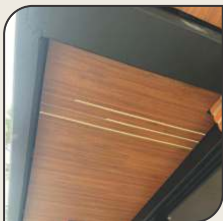
Fita LED embutida no forro
